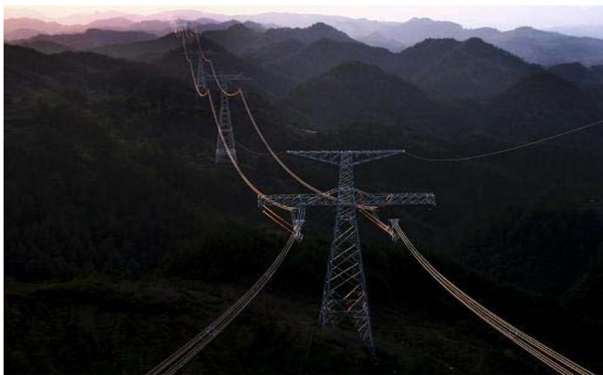
The 800kV HVDC transmission line
